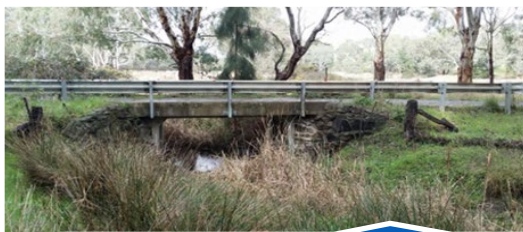
Culverts x 9 (Mont Rosa Bridge - 1981)
