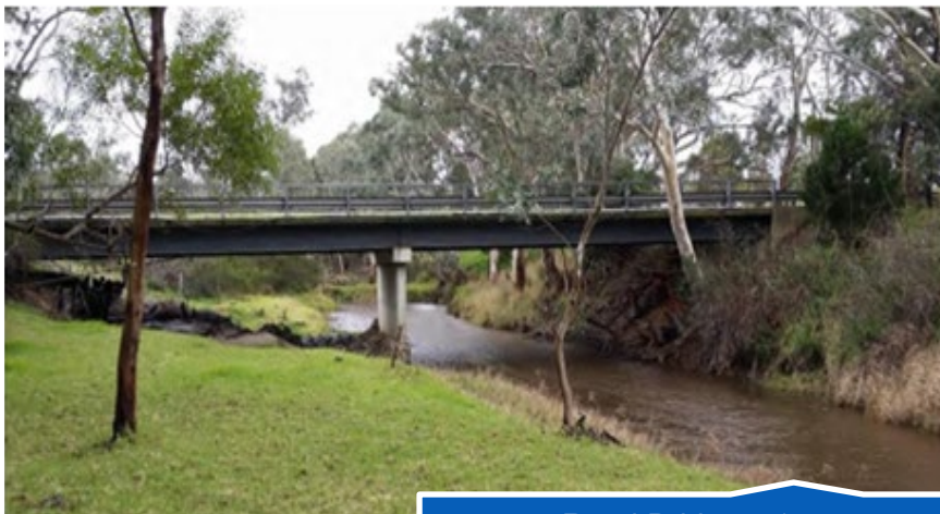
Road Bridge x 15 (Sawpit Road Bridge - 1972)
